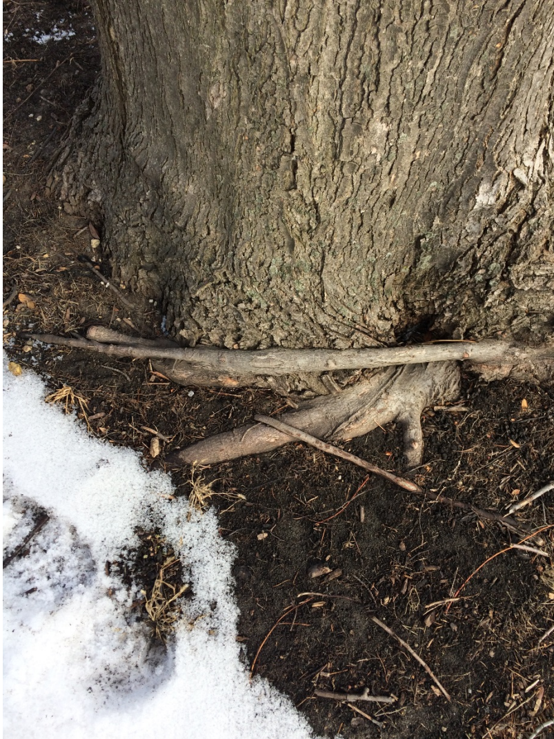
Tree #650 exhibiting girdling roots.
